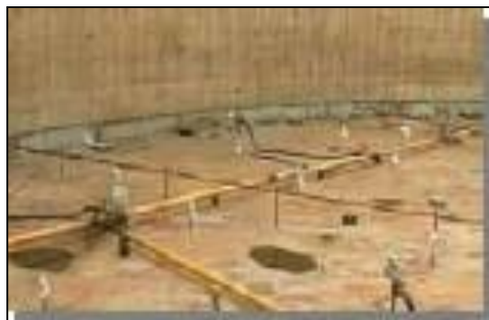
Tank Bottom after application of PC SRS
