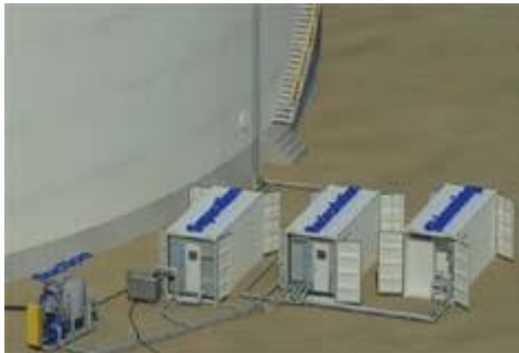
Installation of SRS
